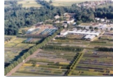
Experimental Station of Ornamental Plants Nowy Dwór Ltd.
